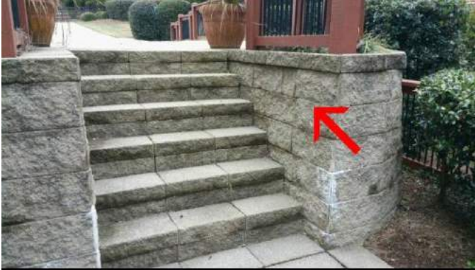
No handrail @ backyard stairs
