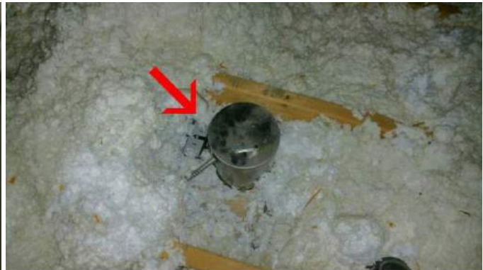
Recessed light in contact with insulation
