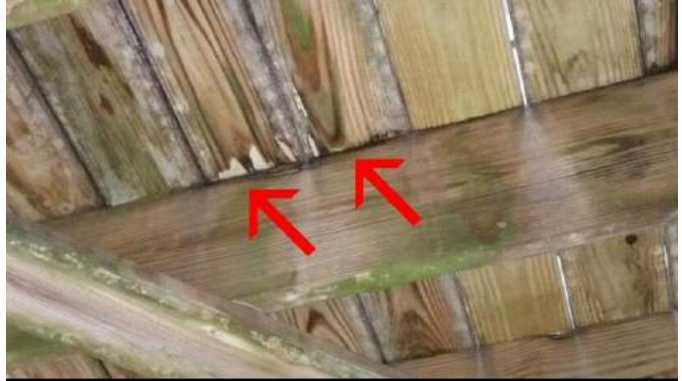
Decay of deck surface boards
