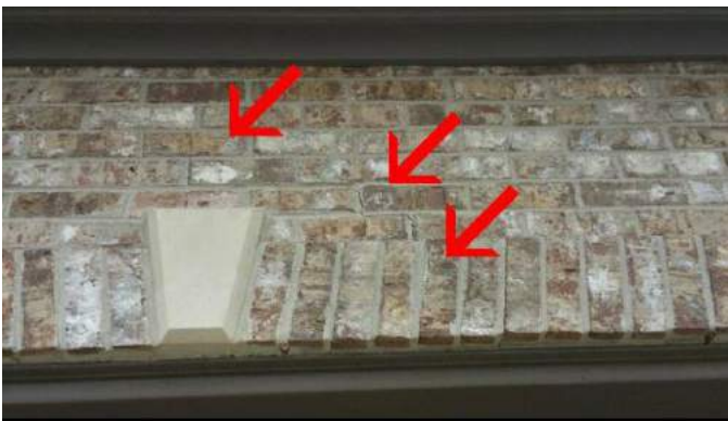
Crack above 2 car garage door
