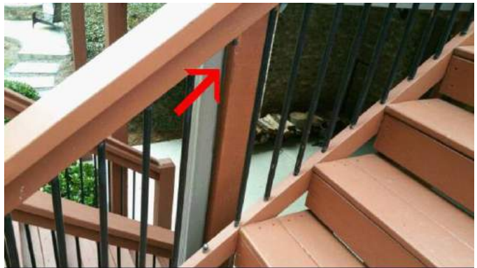
Railing picket is missing
