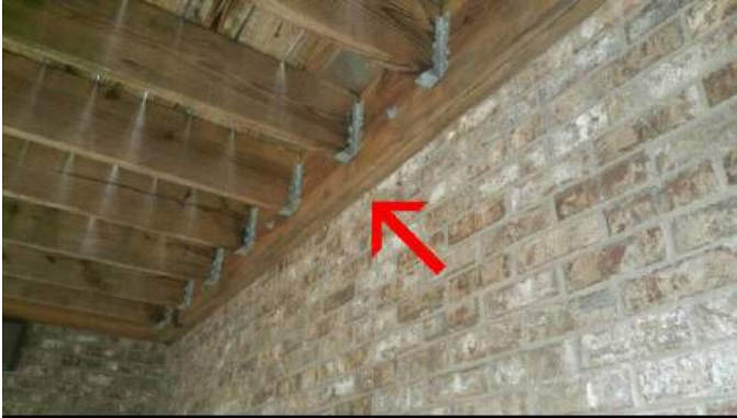
Deck attached over the brick veneer
