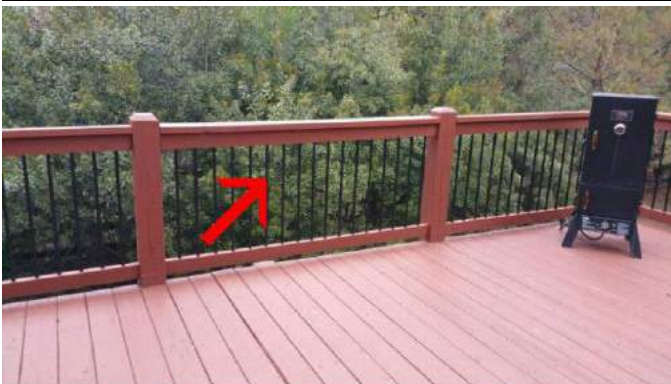
Railing is loose from the deck
