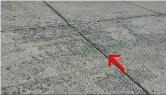
Surface deterioration @ driveway
