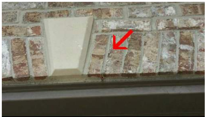
Crack above 1 car garage door
