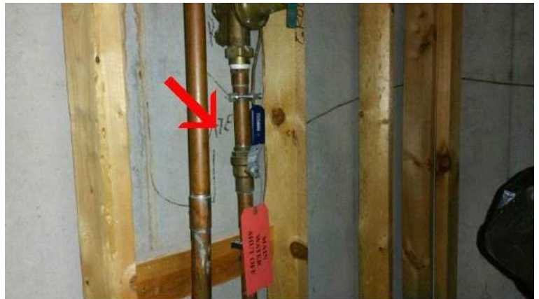
Main water shut off valve
