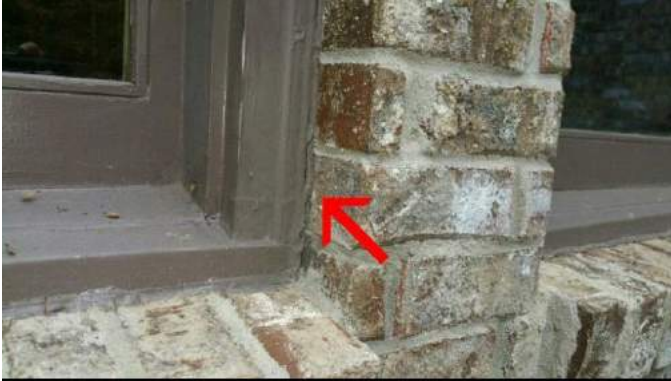
Cracked/loose caulk - rear windows
