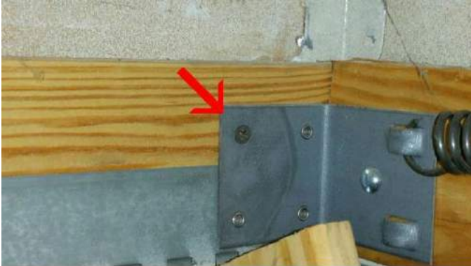
Drywall screws used to secure frame
