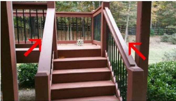
No gripable handrail installed
