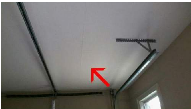
Crack @ 1 car garage ceiling
