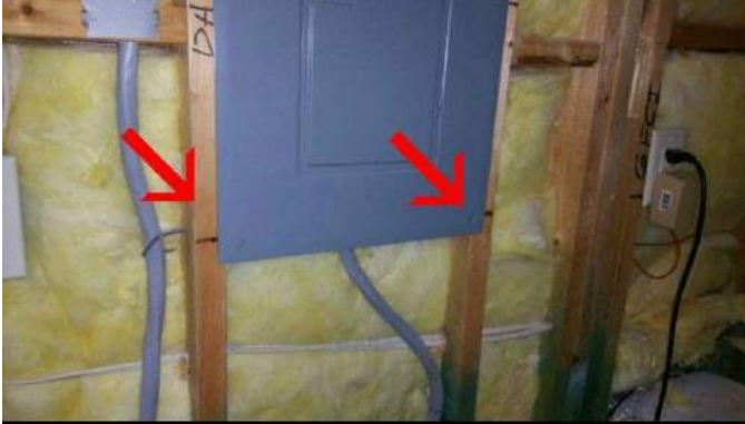
Missing cover screws
